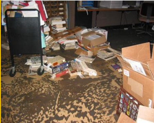
Flood damage at the Gulf Coast Library
